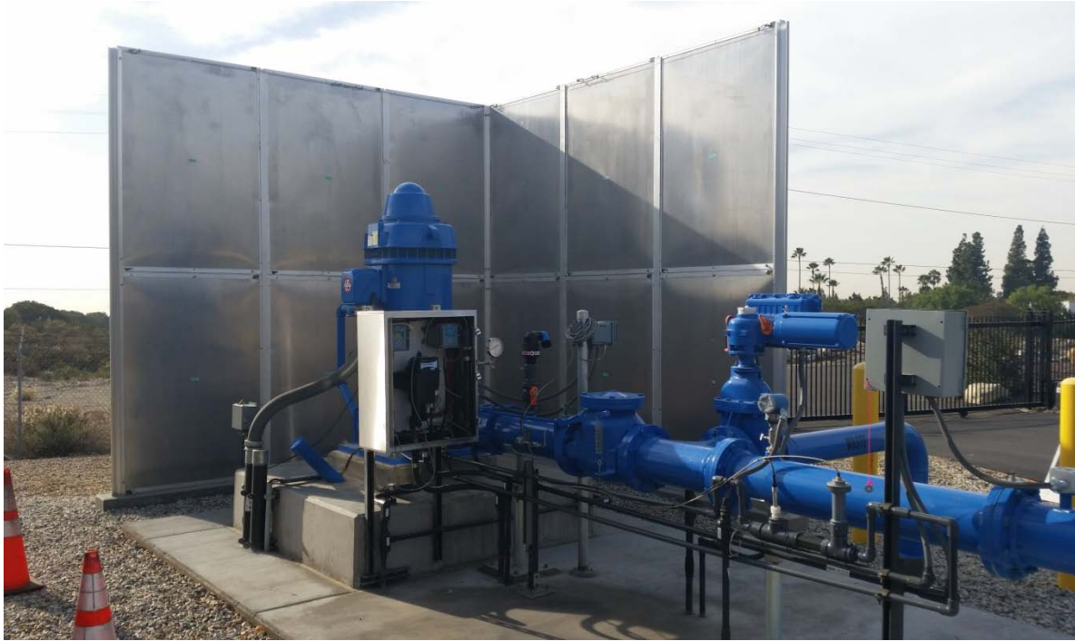
TVMWD Well #2 (completed August 2014)
