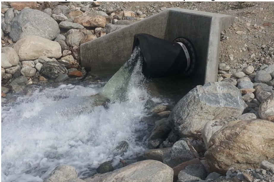
TVMWD Spreading Outlet in San Antonio Spreading Grounds
