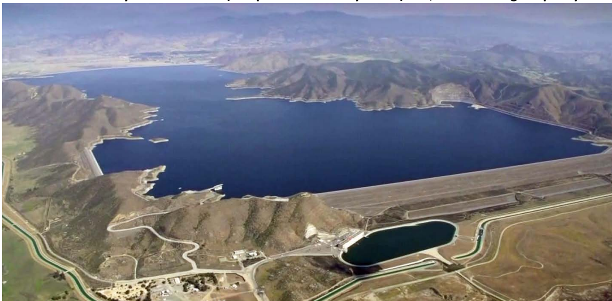
Diamond Valley Lake Reservoir (completed in 2001 by MWD) 800,000 AF Storage Capacity
